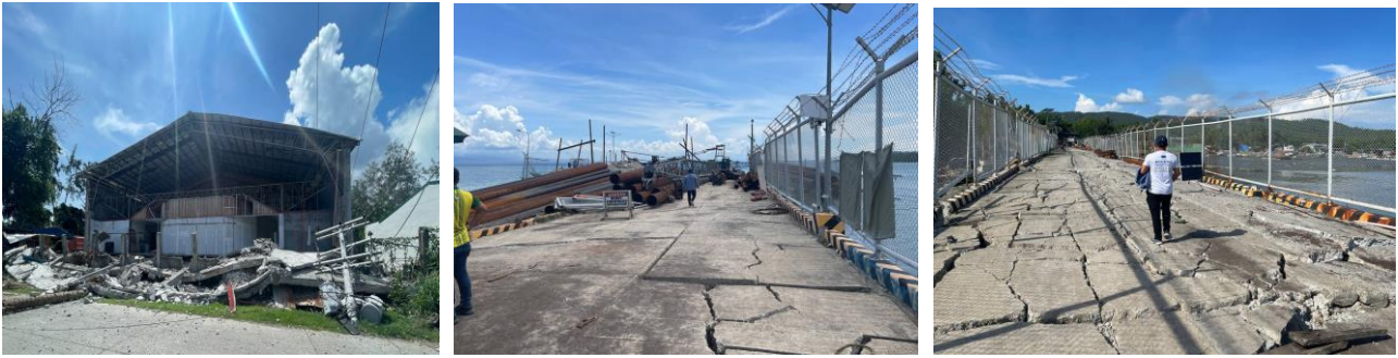
In photos: Inaccessible and destroyed road and infrastructure in the Port of General Santos (Photos by Macy Daproza for Action Against Hunger)
