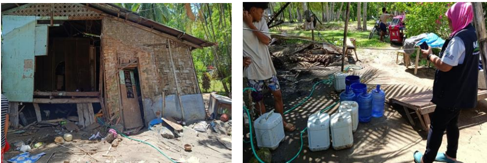
In Photos: (1) Damaged home in Sitio Luot, Barangay Poblacion, Malapatan. (2) Resident showing extent of destruction to Action Against Hunger and MOSEP MERT team. (3) Assessment of water access in Sitio Luot. (Photos by Yasraf Gayao for Action Against Hunger)
